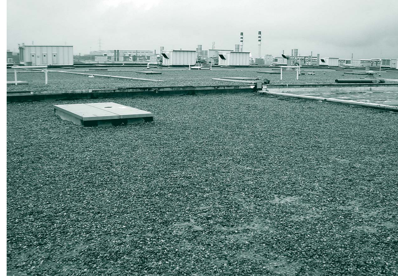
● Fábrica General Motors. Zaragoza . SURE SEAL - 140.000 m 2
