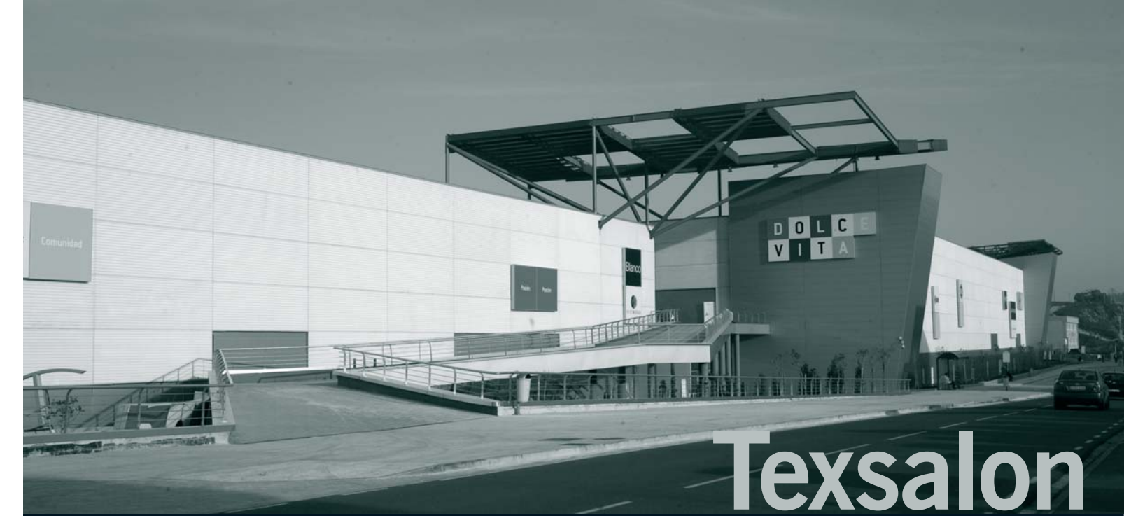
• Dolce Vita Mall. A Coruña (Spain). TEXSALON MP - 45.000 m 2
