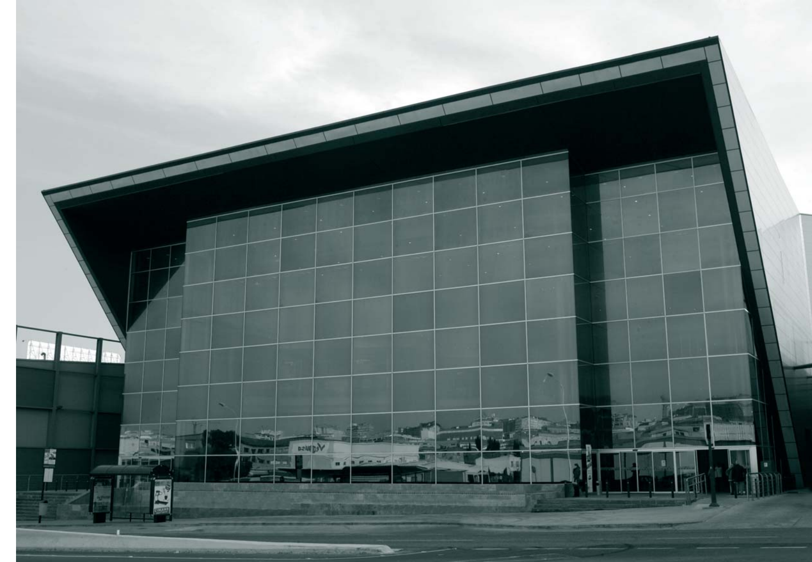
● Dolce Vita Mall. A Coruña (Spain). TEXSALON MP - 45.000 m 2
