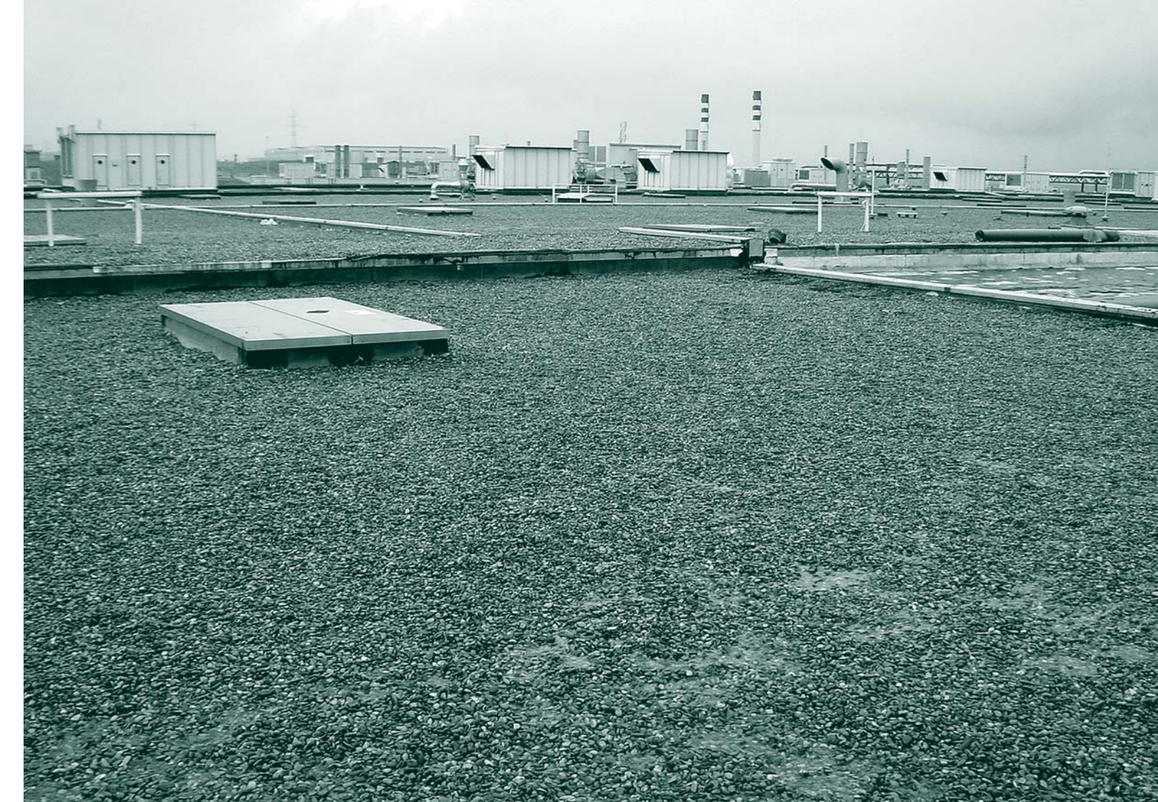
● Fábrica General Motors. Zaragoza . SURE SEAL - 140.000 m 2
